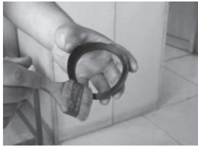
2. Spread lubricant on gasket ring.
