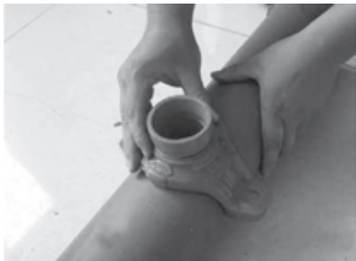
4. Install the Mechanical Tee in the hole.
